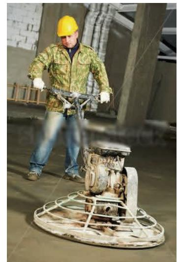
*Machine-troweled concrete is an example of a smooth floor.*
